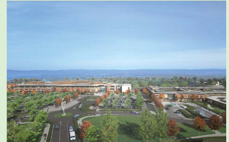
Above: An aerial view of the New Omagh Hospital Complex
