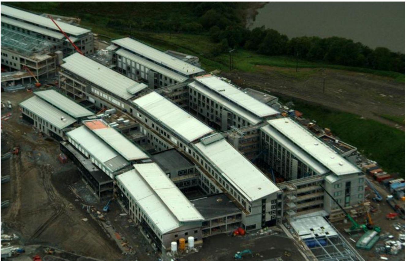
Photograph 4: Metal Roofing nearing completion in several blocks (September 2010)
