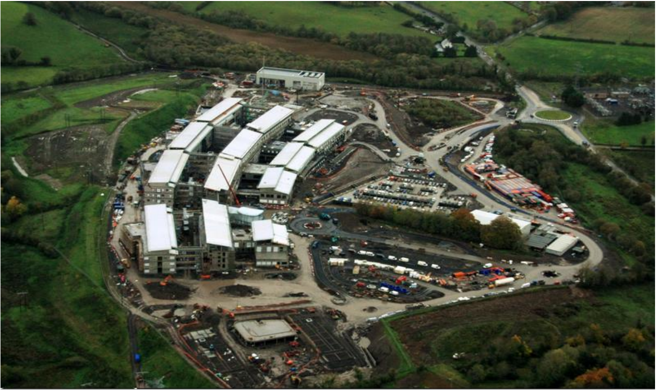
Photograph 10 – South Elevation Overview (October 2010)
