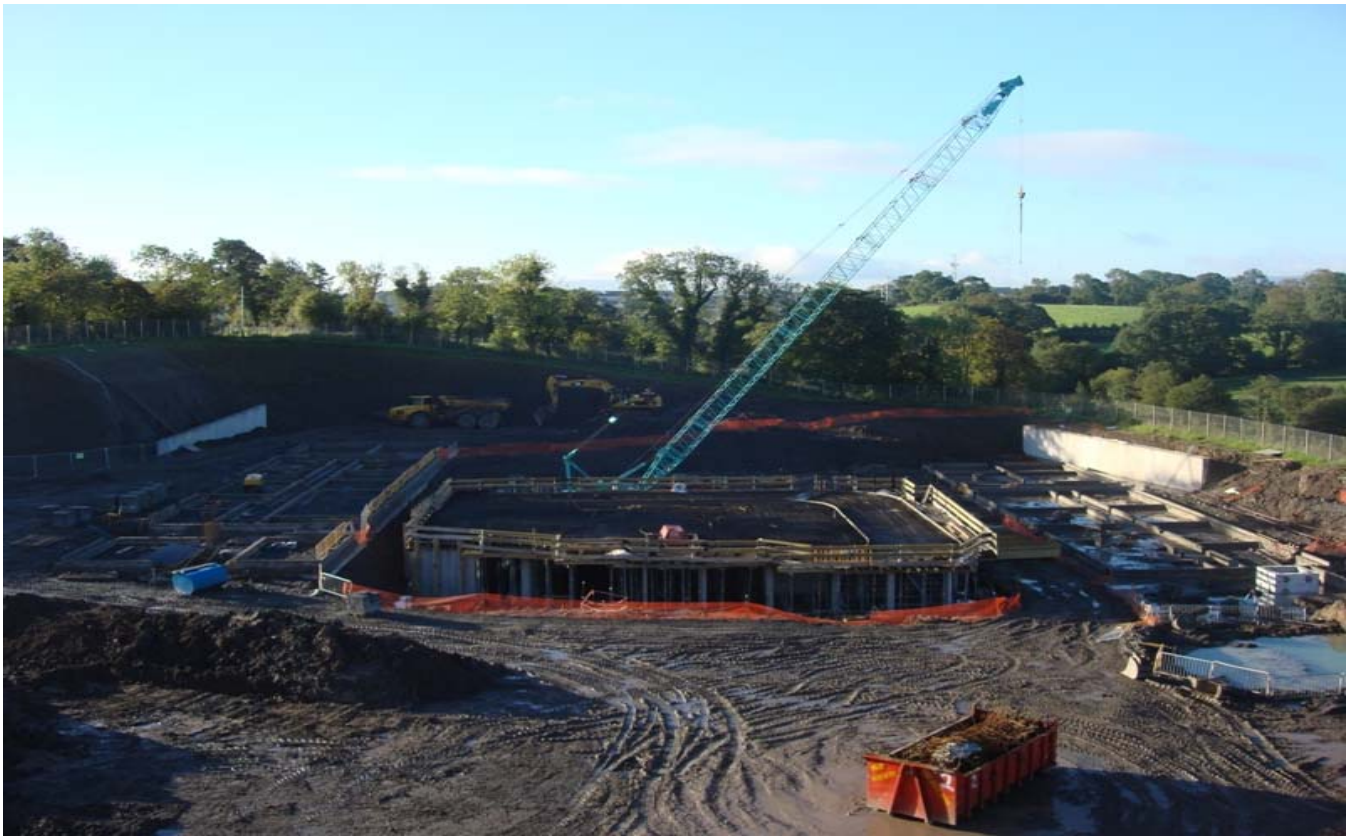
Photograph 5: Substructure works nearing of completion to KWA (September 2010)
