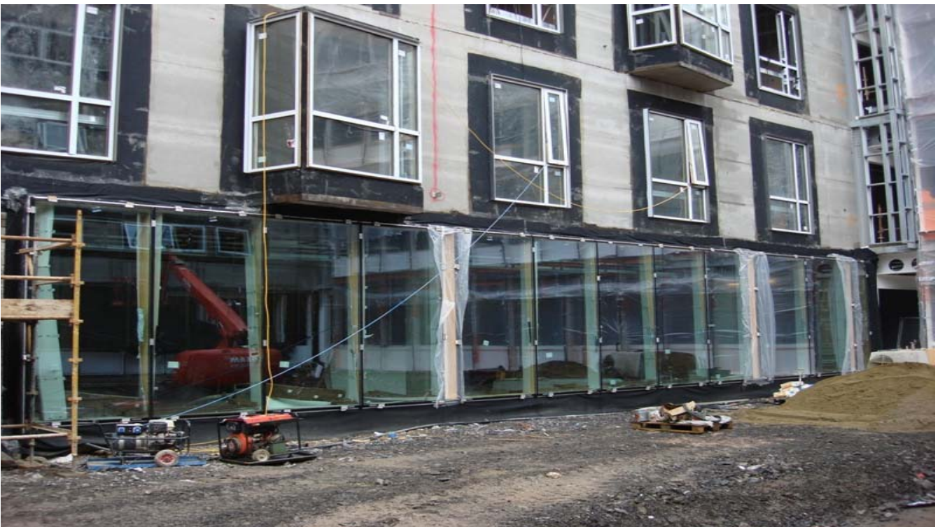
Photograph 11 – Hospital Street Curtain Walling (October 2010)
