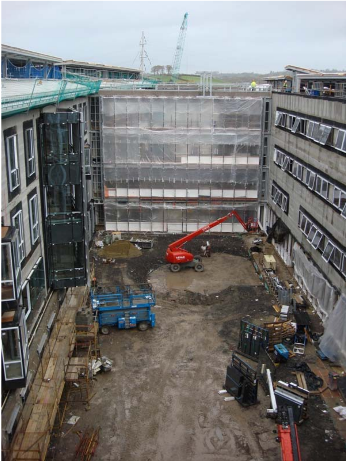
Photograph 12 – Link Bridge – Curtain Walling (October 2010)
