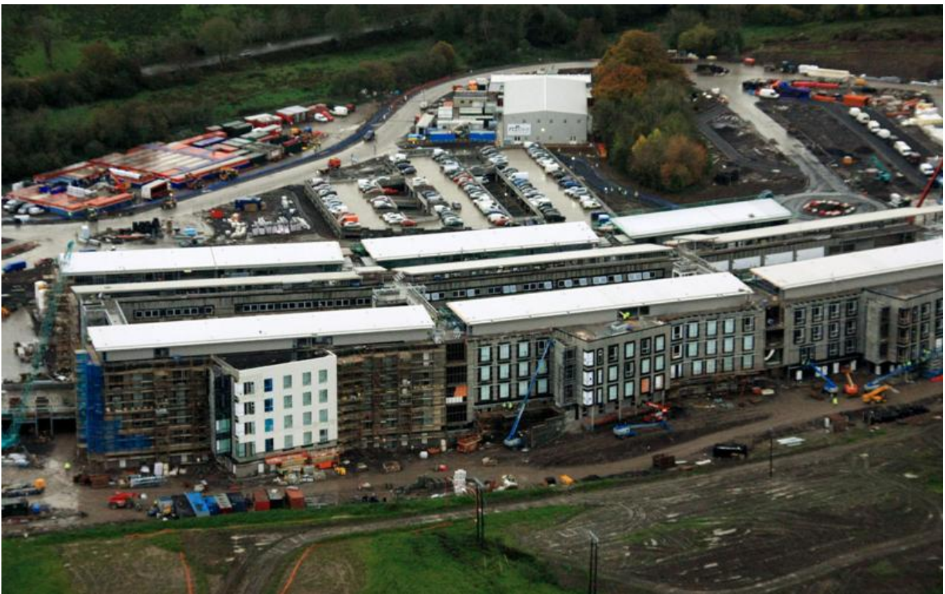
Photograph 9 – West Elevation Overview (October 2010)
