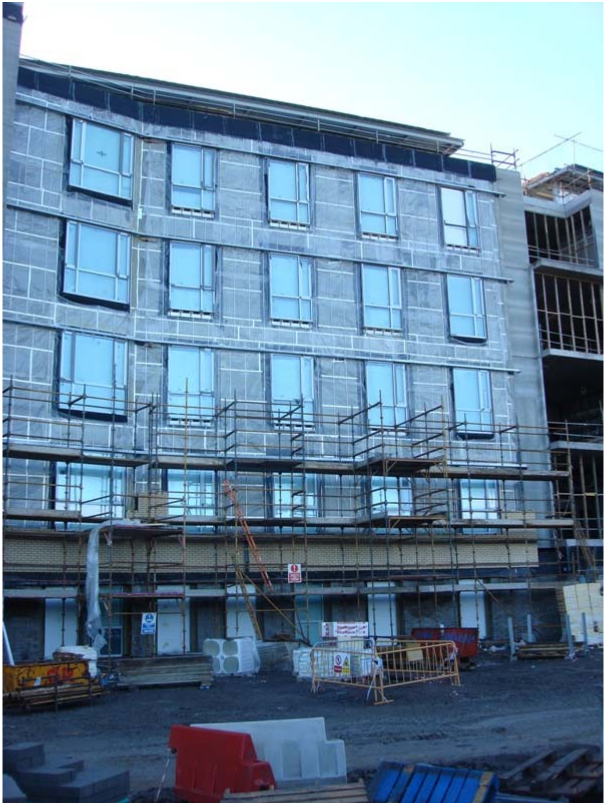
Photograph 7: Brickworks progressing in Elevation 2 (September 2010)
