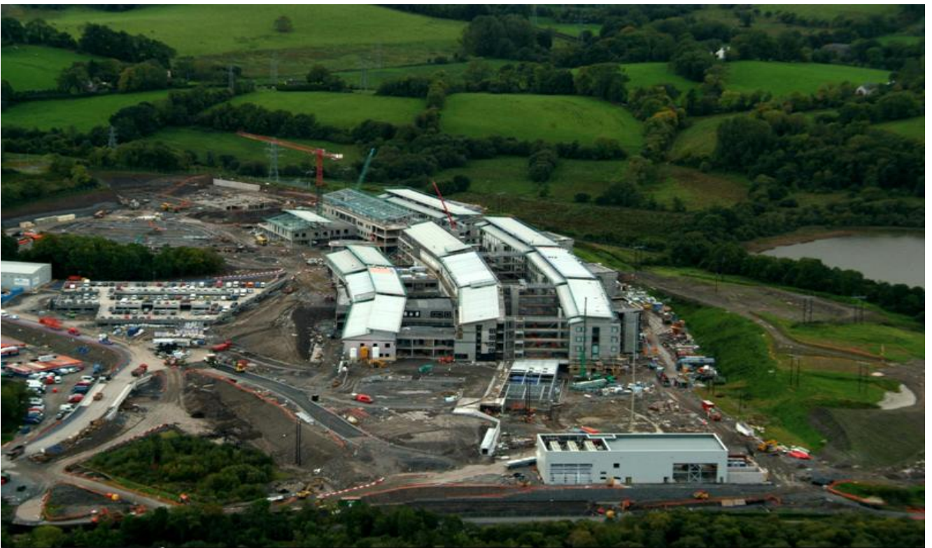
Photograph 2: Energy Centre and North Elevation Overview (September 2010)
