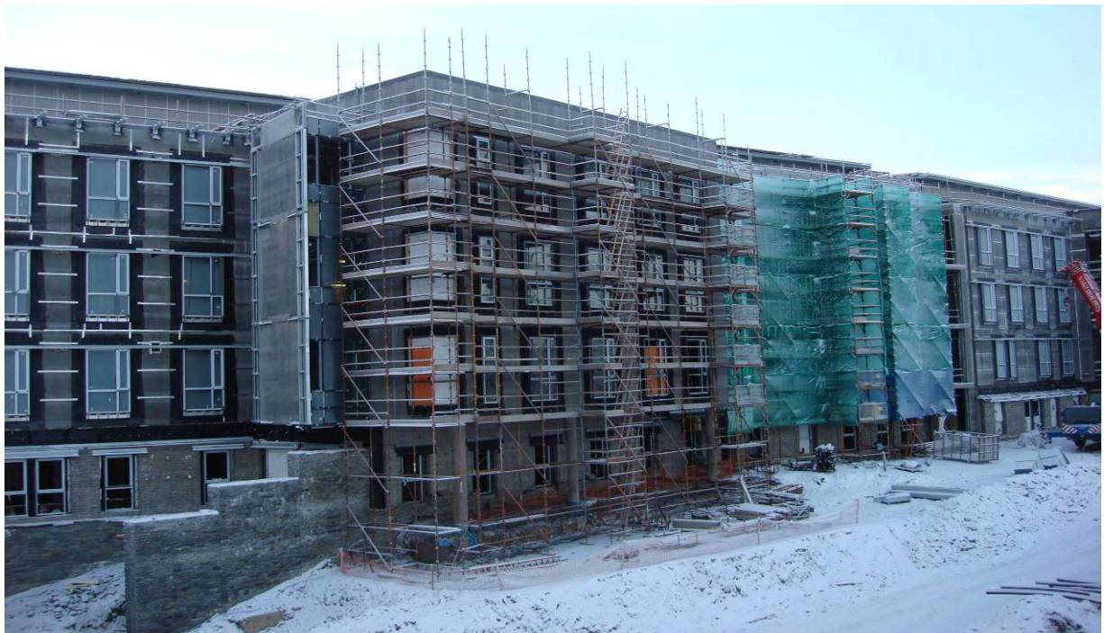
Photograph 2 – Block F and D West Elevation Overview. Inclement weather conditions (November 2010)
