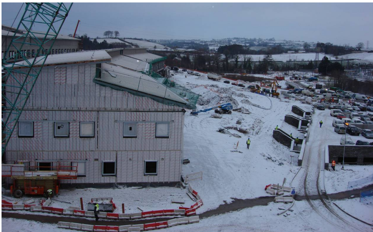
Photograph 4 – Block E Façades works. Inclement weather conditions (November 2010)
