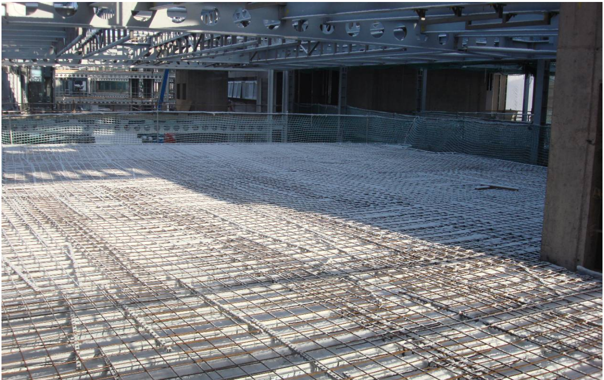
Photograph 9 – Block C Slab level 1. Inclement weather conditions (November 2010)
