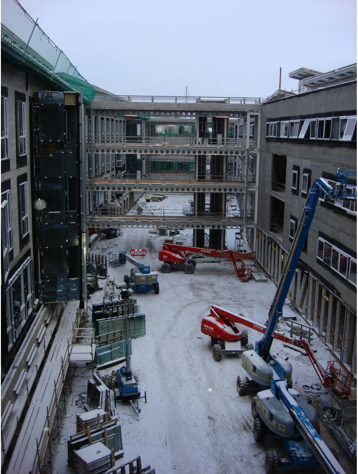
Photograph 5 – Link Bridge 4. Inclement weather conditions (November 2010)
