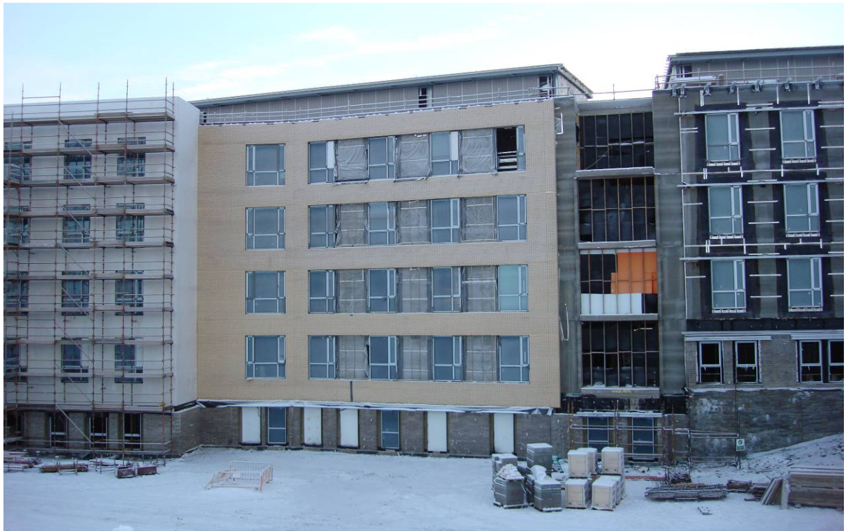
Photograph 1 – Block H West Elevation Overview. Inclement weather conditions (November 2010)
