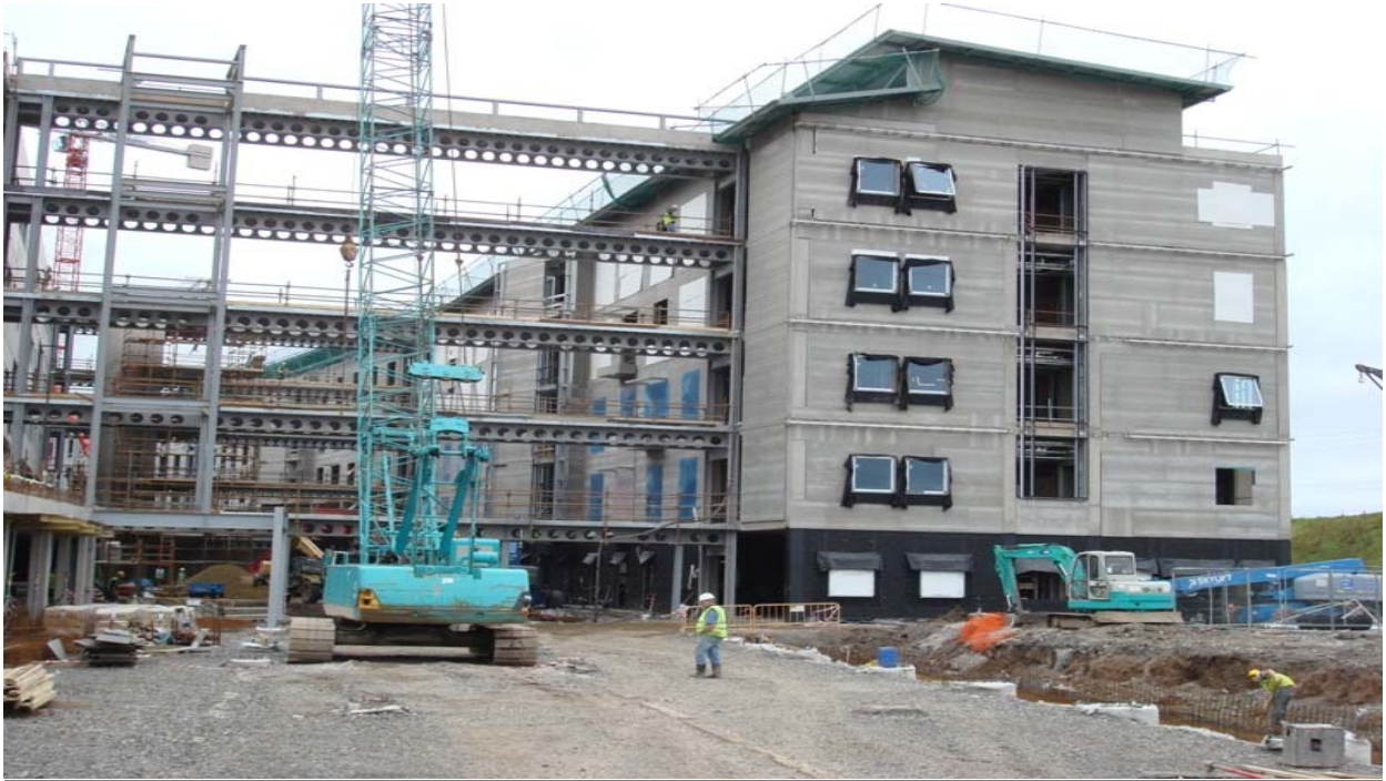
Photo 5 – Link Bridge 5 Completed & Substructure Works in Laundry
