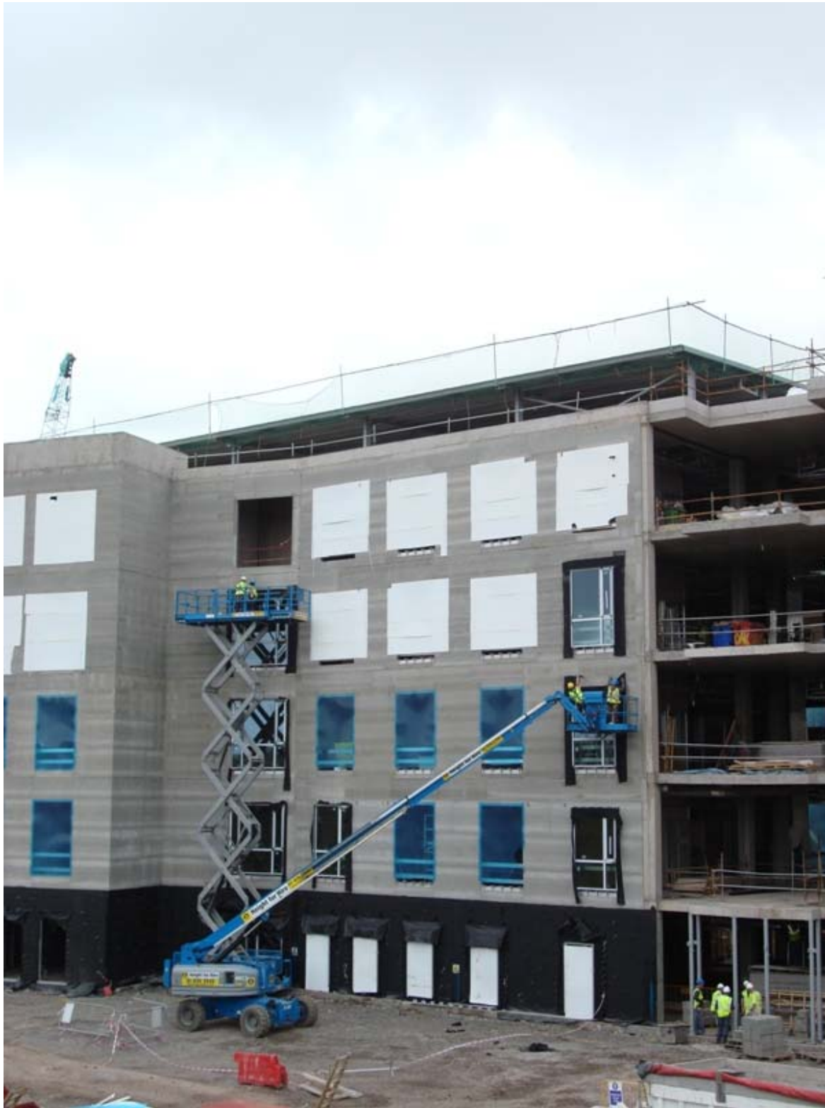
Photo 7 – Installation of Windows
