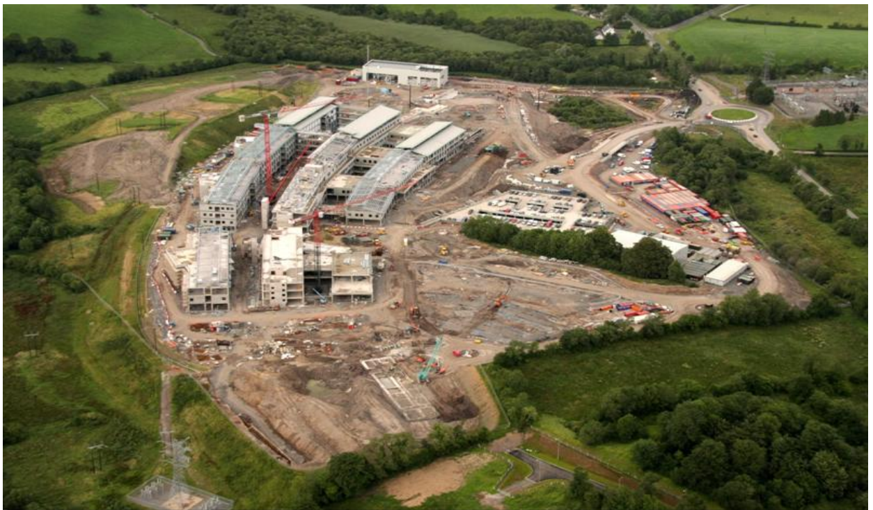
Photo 4 - Site Overview (Taken from KWA)
