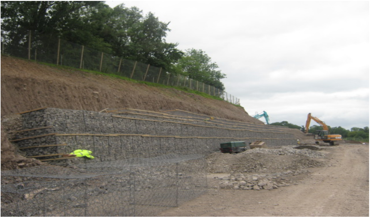
Photo 6 – Gabion Walls nearing completion in front of South Car Park
