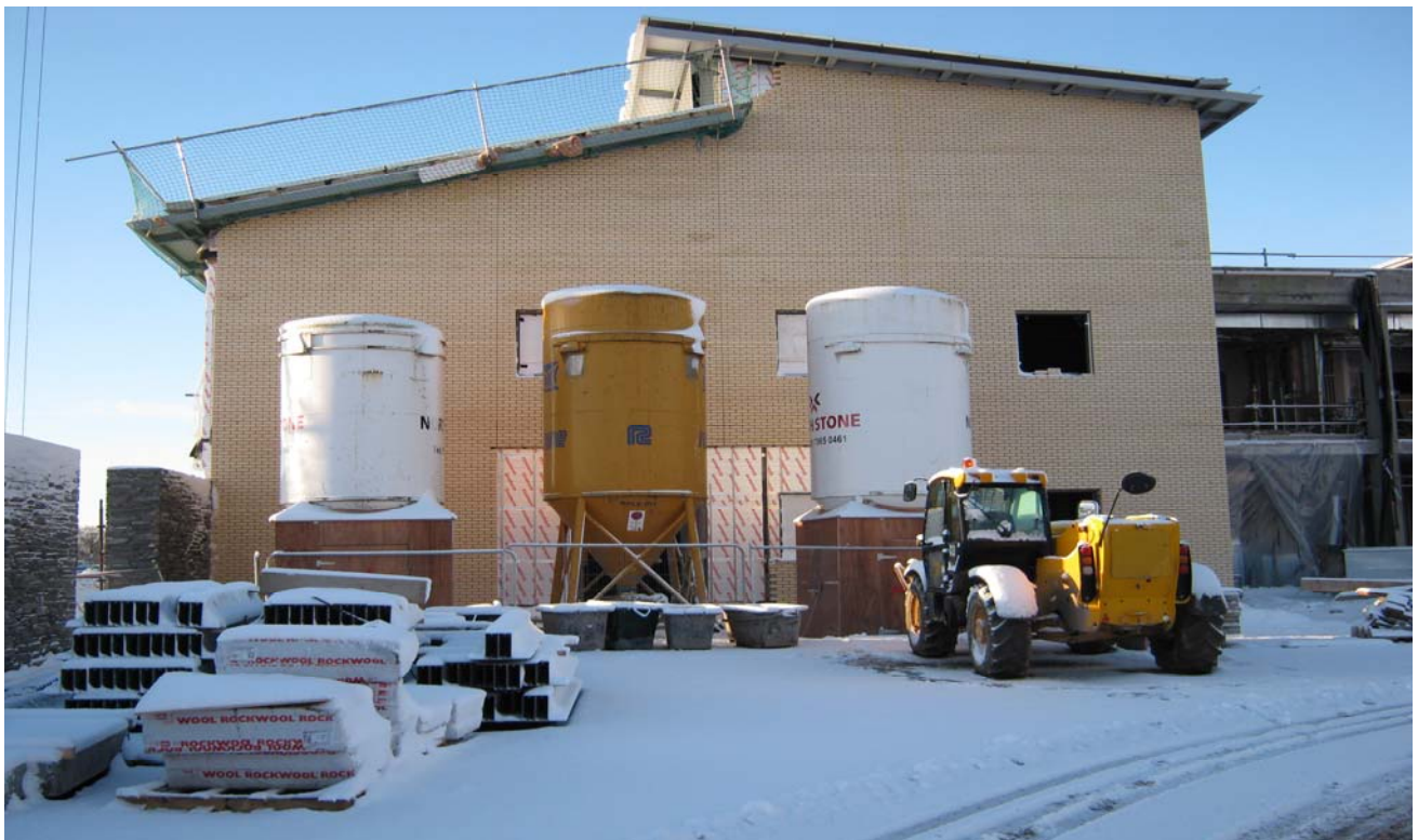
Photograph 2 – North Elevation (December 2010)
