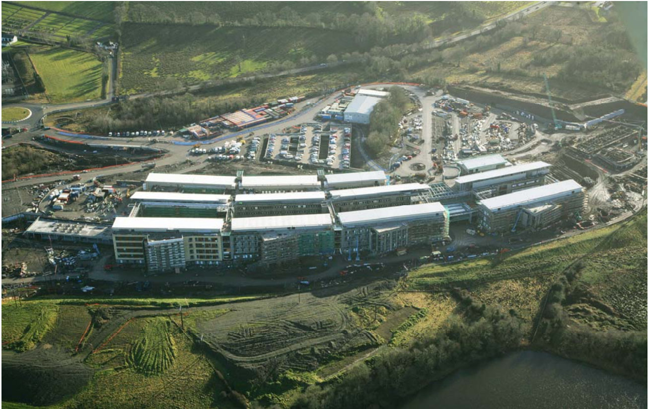
Photograph 3 – West Elevation (January 2011)
