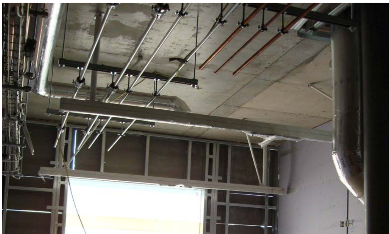
Photograph 12 – Into Some Rooms on Block H, commencement of hoist installation
