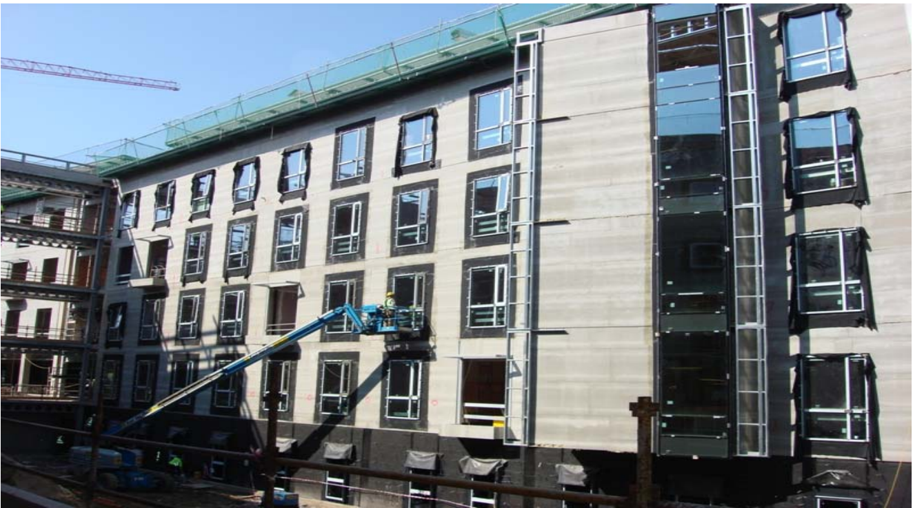
Photograph 10 – Windows & Curting Walling Installation nearing completion for Elevation 28 on Block H
