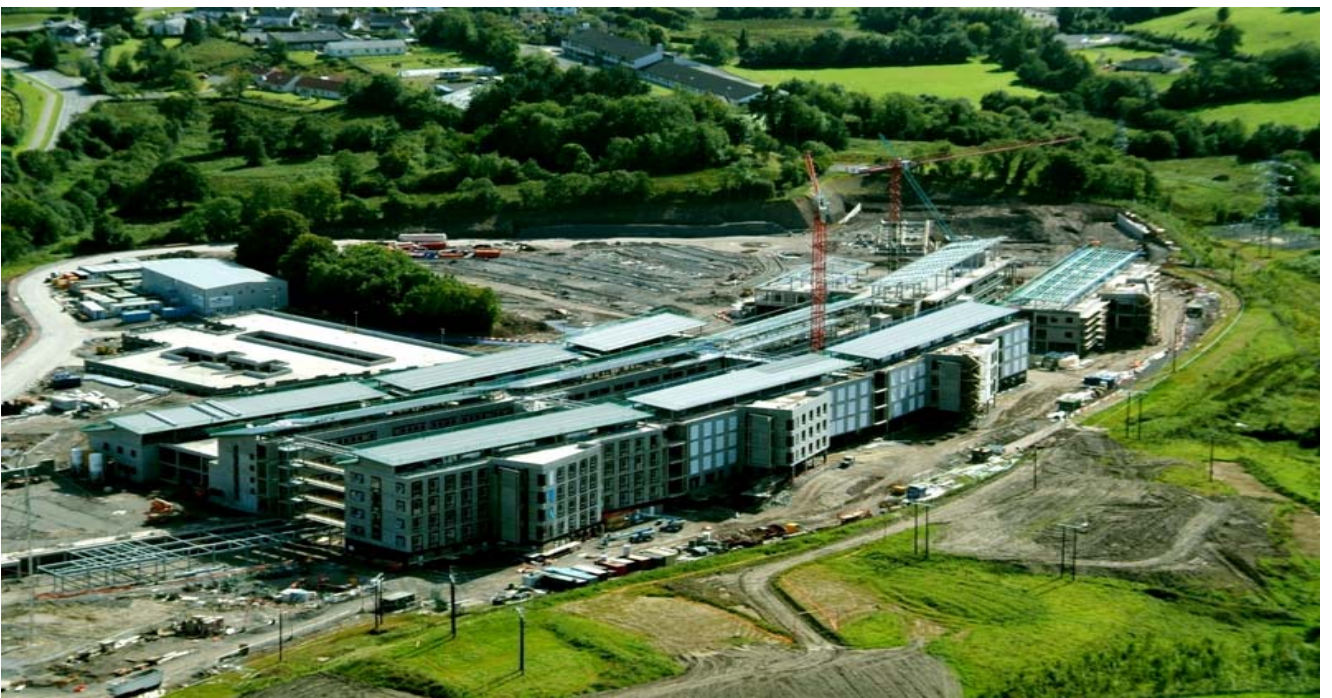
Photograph 2 – West Elevation Overview taken from West Meadow
