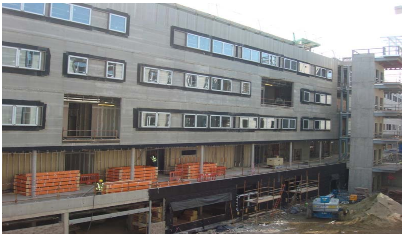
Photograph 11 – Duda-Block J Elevation to Linear Garden
