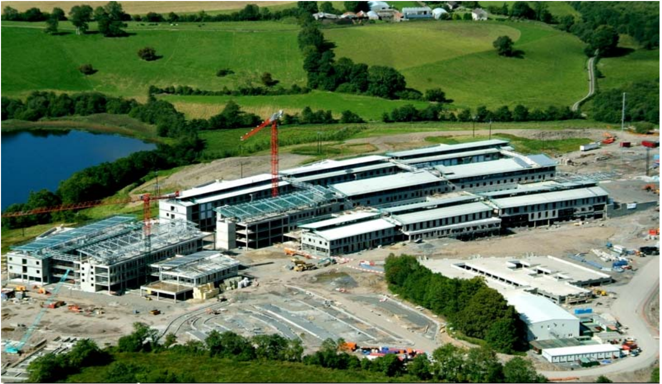
Photograph 3 – East Elevation Overview
