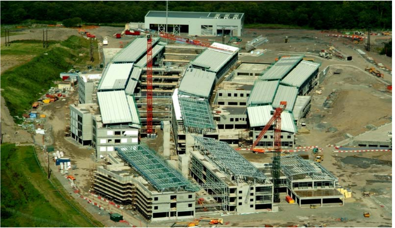
Photograph 5 – Roofing Works. Lining sheet nearing completion in several blocks
