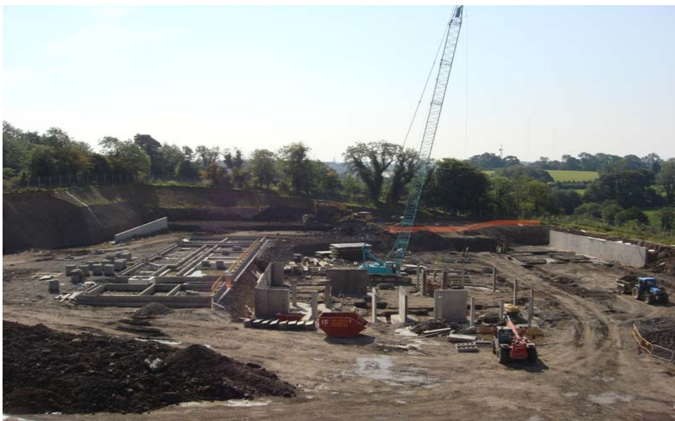
Photograph 8 – KWA from Plantroom ob Block B3
