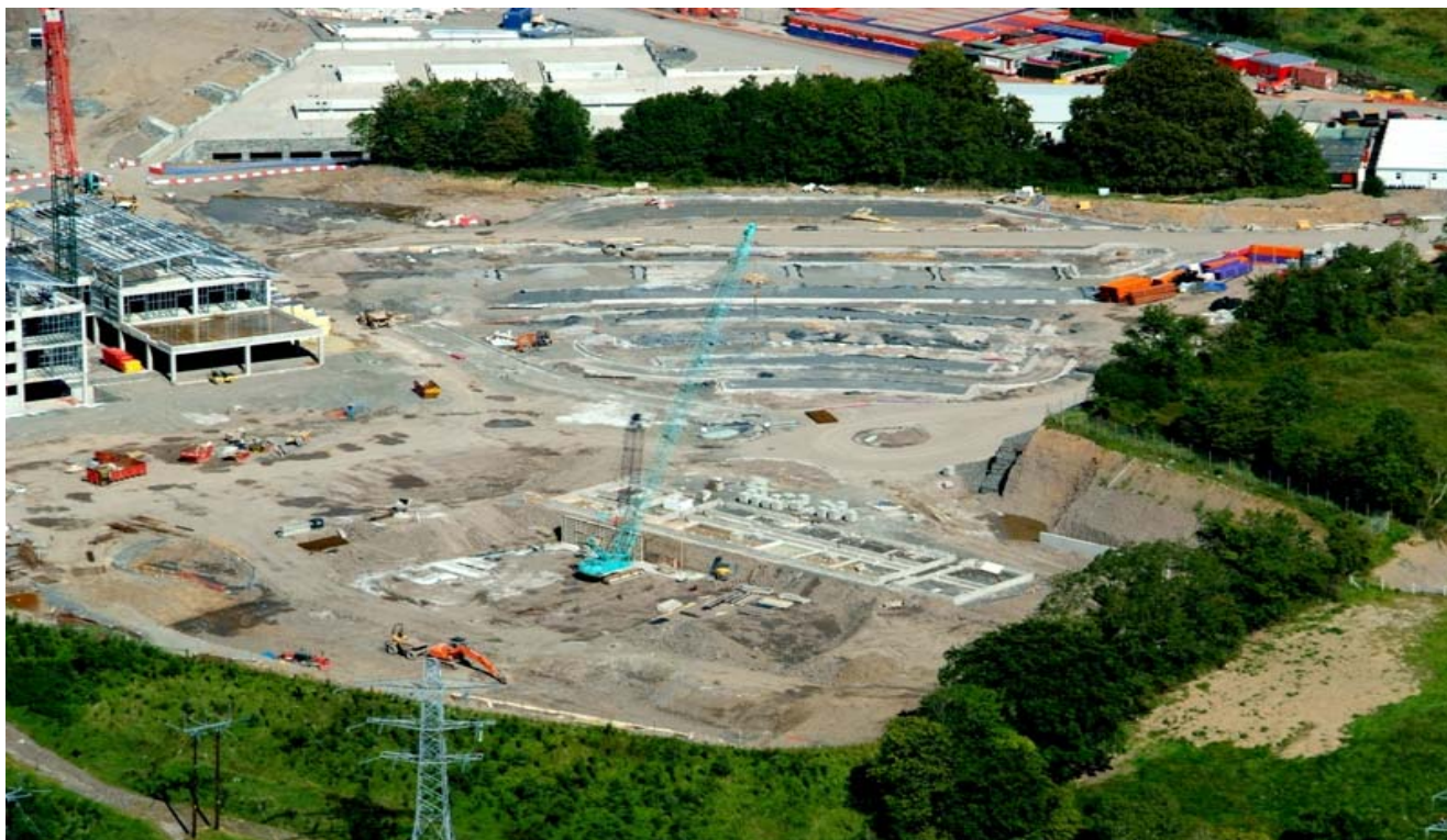
Photograph 7 – KWA and South Car Park Overview
