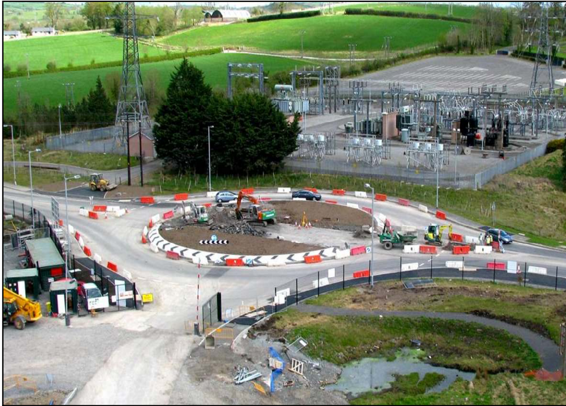
Photo 7 – Main Entrance Roundabout works Nearing Completion
