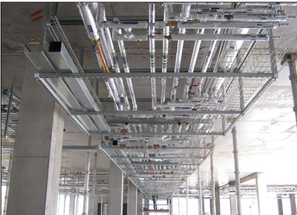
Photo 6 – Clinical Block M&E Installations Progressing
