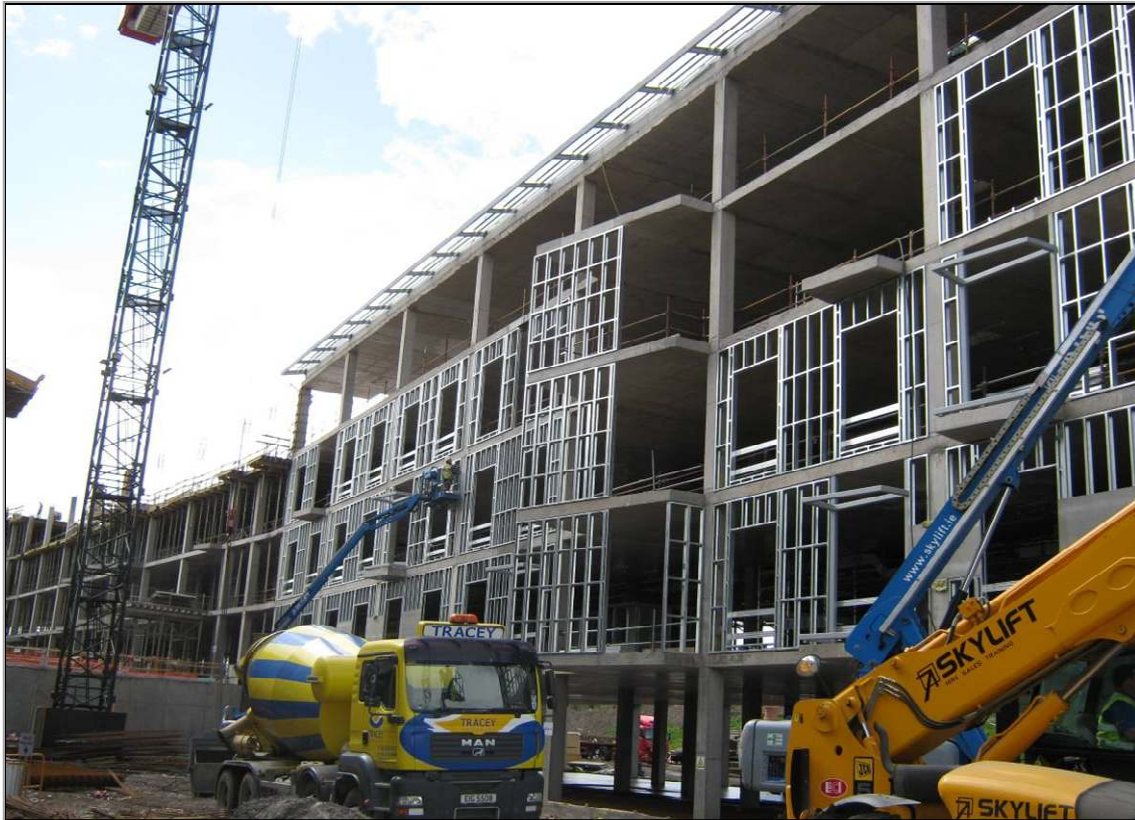
Photo 4 – Ward Block Envelope Progressing
