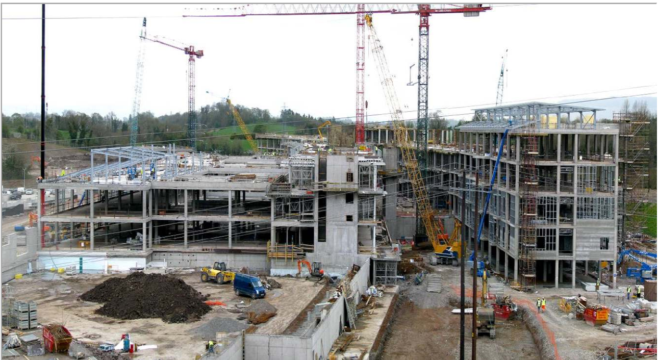
Photo 8 – Steelwork Progressing to Ward & Clinical Block Plantrooms
