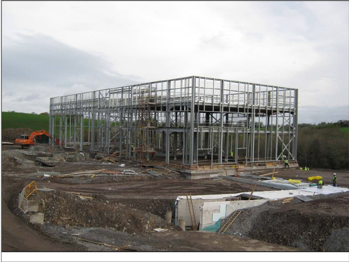
Photo 3 – Energy Centre Superstructure Now Complete
