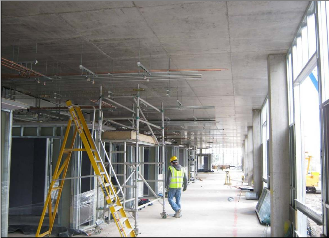
Photo 5 – Ward Block Internal Finishes Progressing
